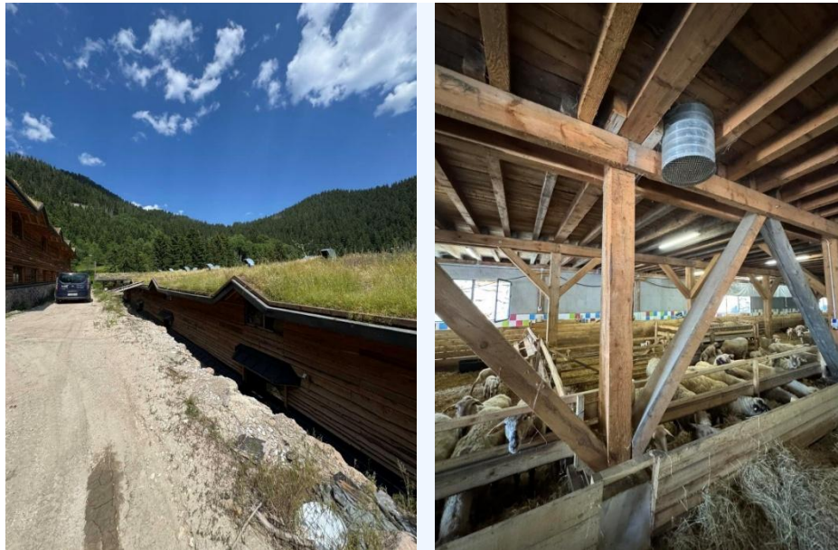
Fig. 3. Photos of barn 1 – outside (left) and inside (right).
